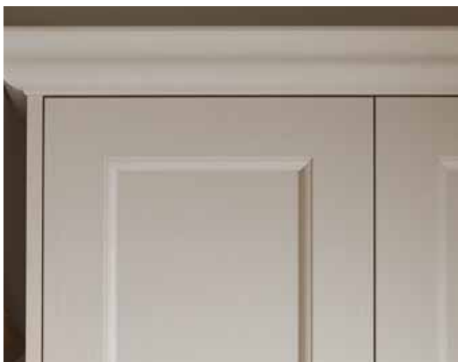
An elegant quarter round bead offers an extra level of detail
